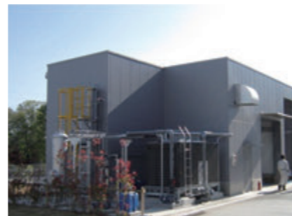
The Tokyo Plant water treatment facility
